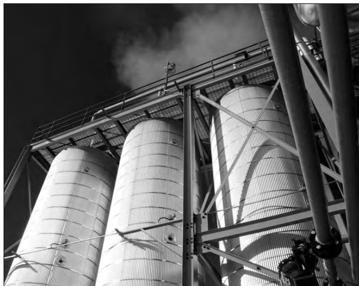
Ethanol Plant Photo: Aaron Brown
