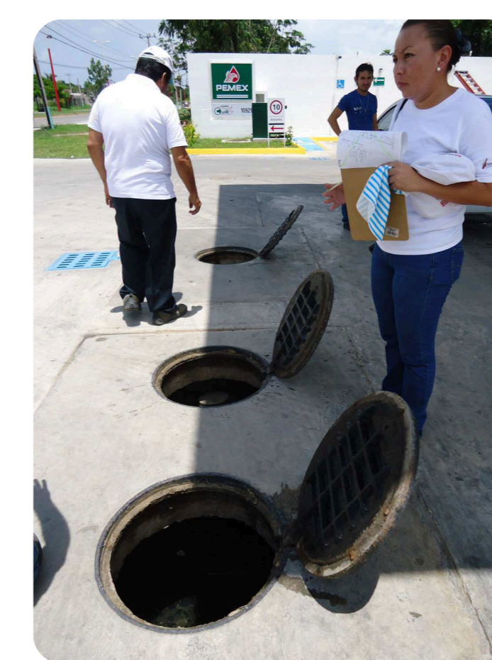
Fuel station inspection. Diego Cano
