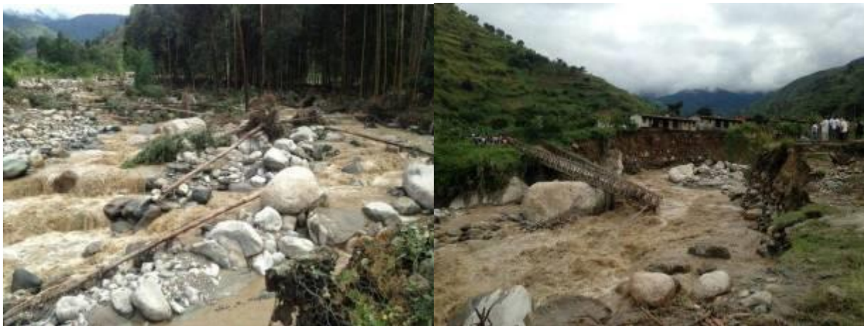
Figure 22: Impact of floods on biodiversity and local infrastructure in Kasese district (Source: CCU File Photos 2013)
