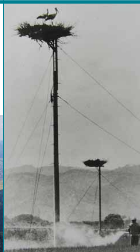
(Photo courtesy of Kobe Shimbun)
